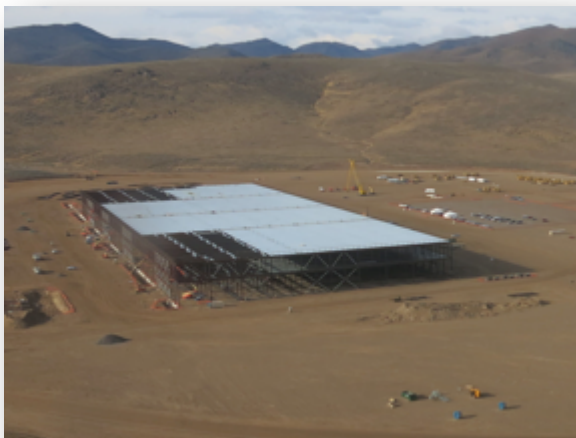
Gigafactory Construction Progress
